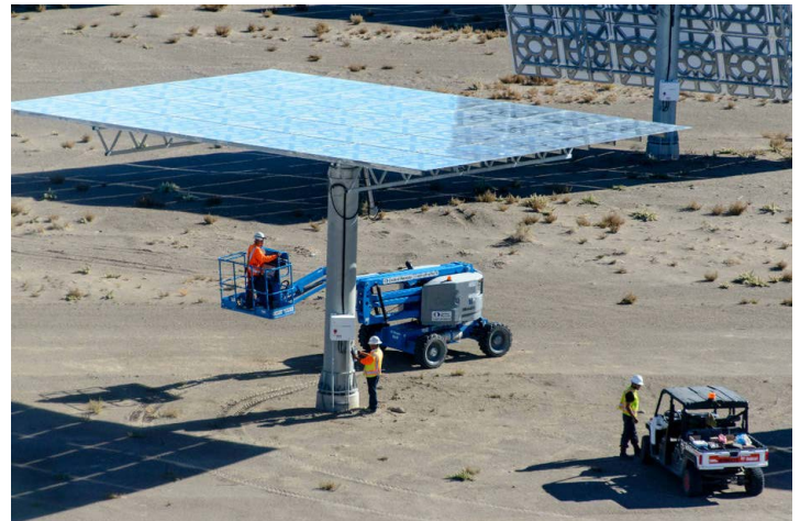
Heliostats, the giant mirrors that focus the sun's rays, are directed by software that allows them to follow the sun through the day. Credit: SolarReserve
