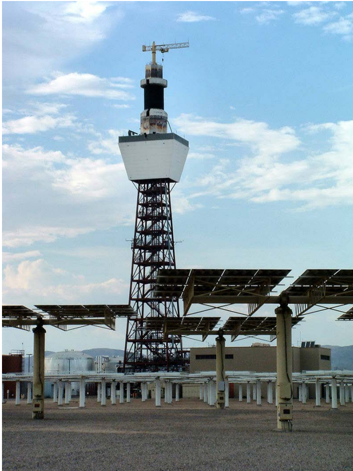
Solar Two was a small pilot project near Barstow, California, where salt storage technology now used at Crescent Dunes was tested in the 1990s. Credit: KJKolb/CC-BY-SA-2.0
